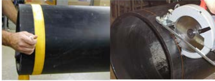
Figure 5: Marking and cutting larger diameter pipes
